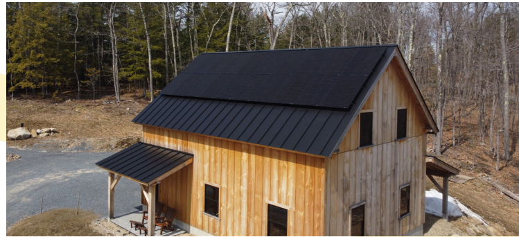
Another PAREI member adds solar to their home: 8.7kW PV array, October 2025
