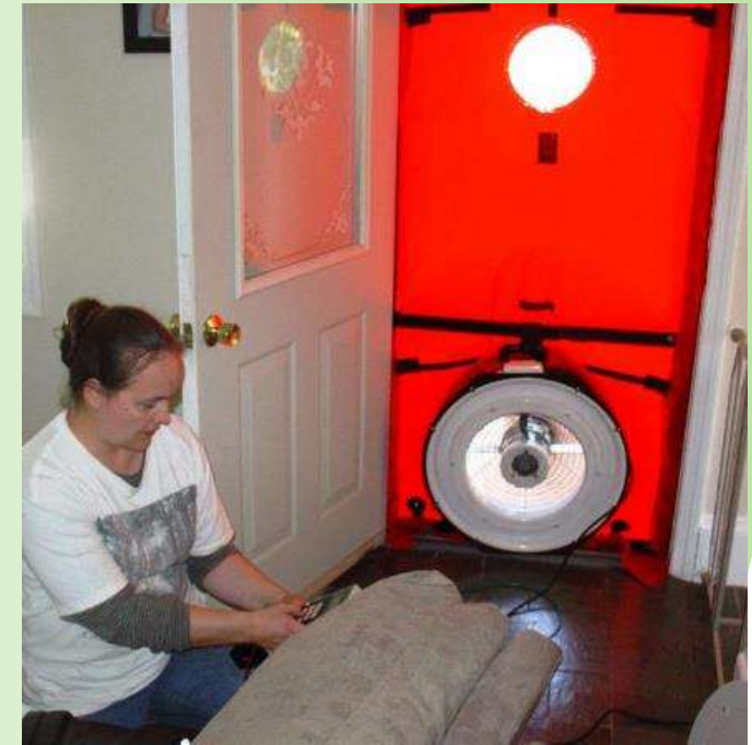
Blower door tests now Energy Code-required
