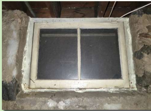
Around old basement windows
