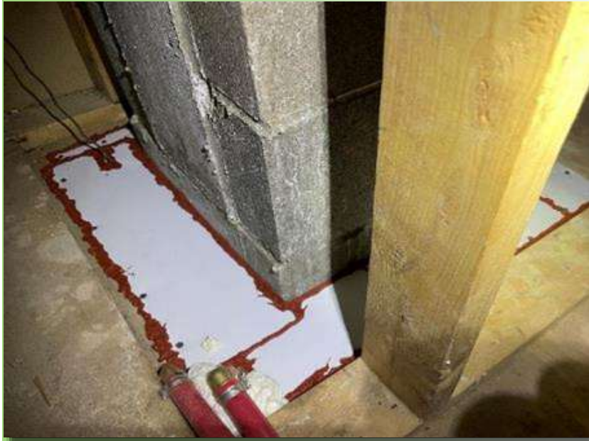
Air sealed chimney chase w- fire-rated materials
