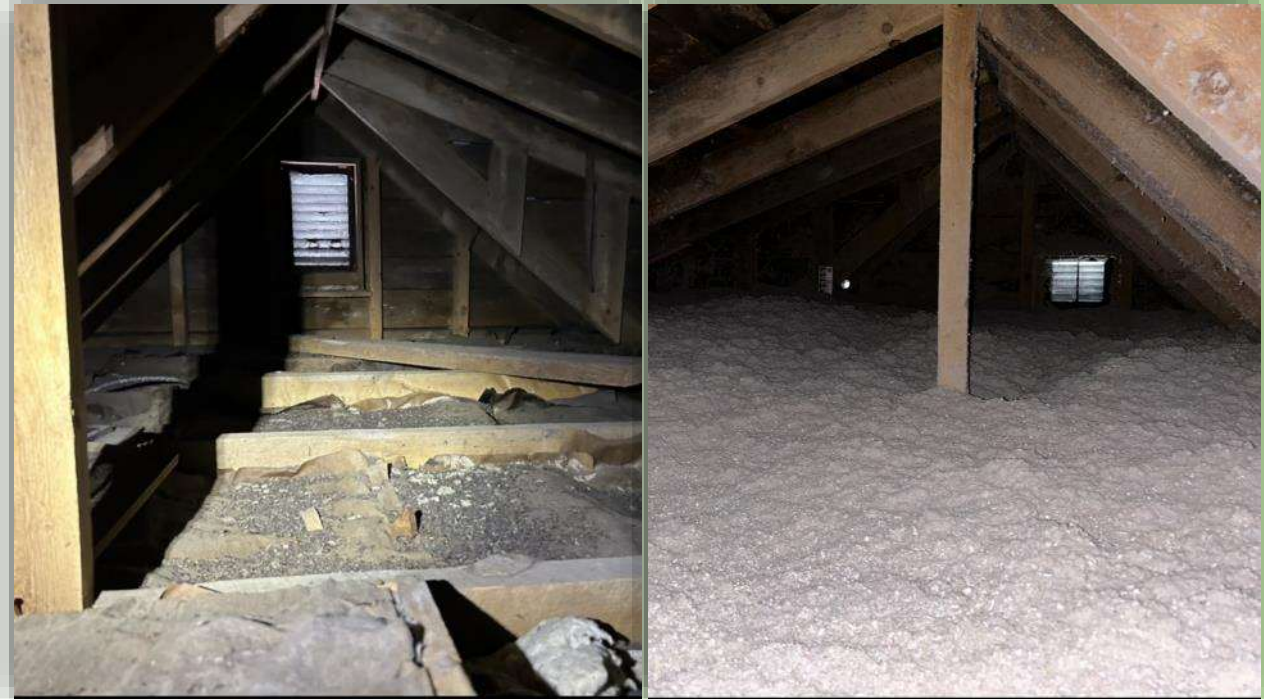
Attic before and after air sealing & insulation
