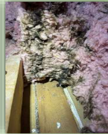
Tops of interior walls
