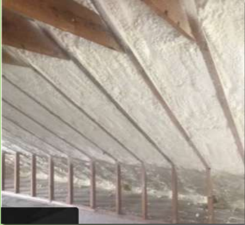
Spray foam prior to drywall fire barrier
