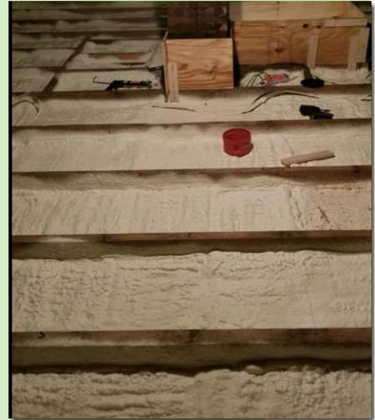
Spray foam "skim coat" attic air seal, prior to insulation
