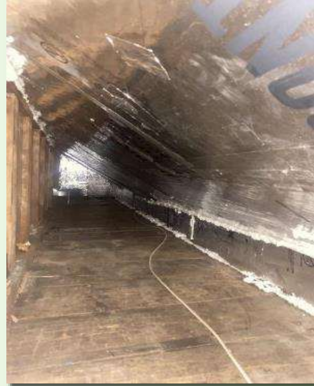
Metal-faced "Thermax" brand foam board is fire-rated for kneewalls
