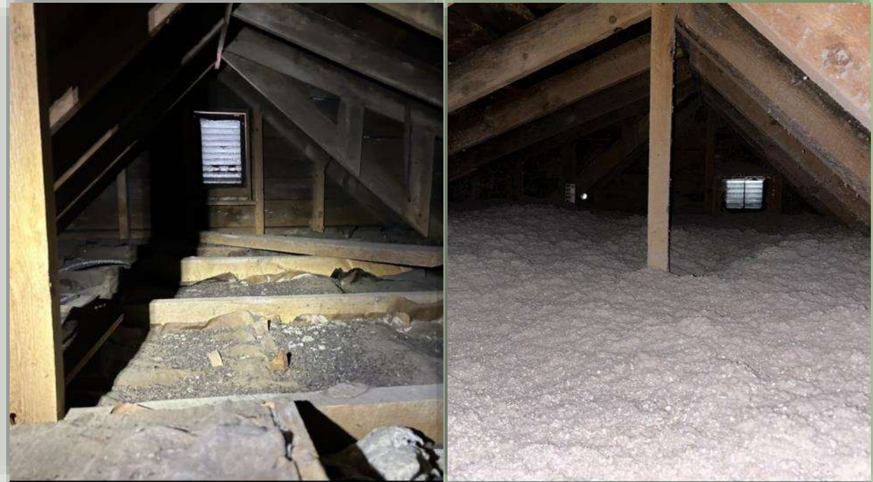
Attic before and after air sealing & insulation
