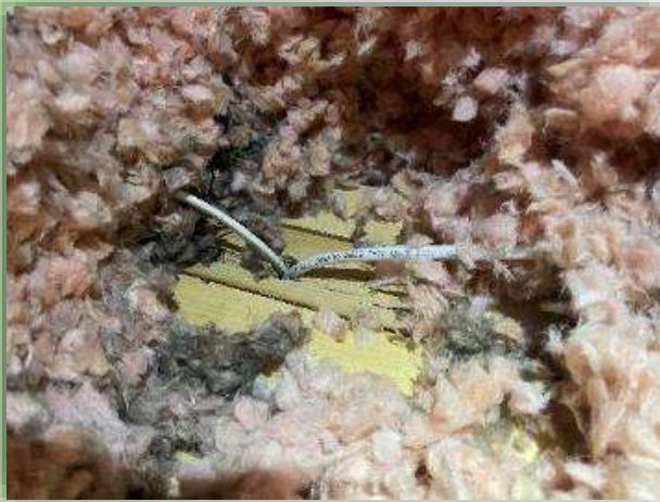
Pipe & electrical penetrations
