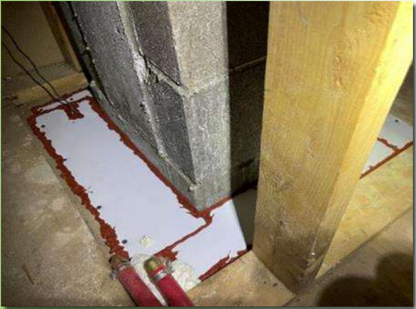
Air sealed chimney chase w- fire-rated materials
