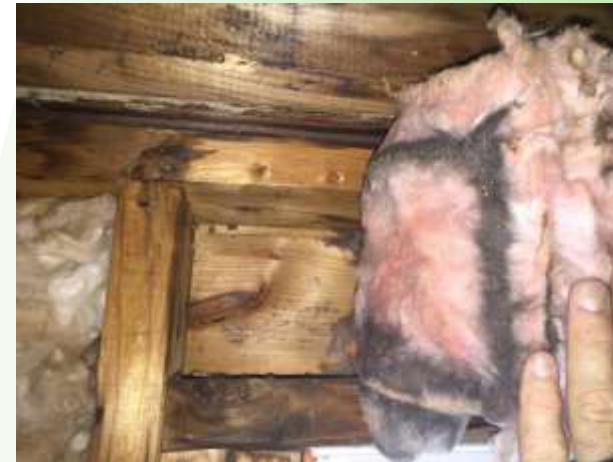
Stained “filter-glass” from air leakage
