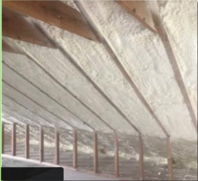
Spray foam prior to drywall fire barrier
