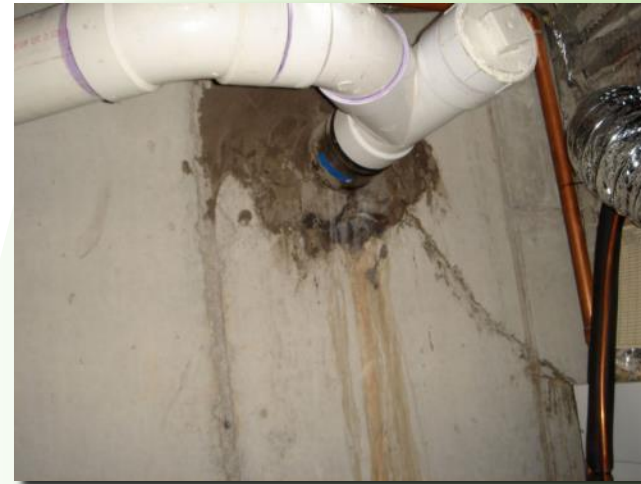
Electrical, plumbing and other penetrations
