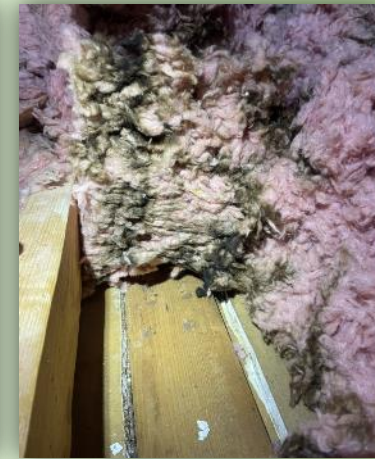
Tops of interior walls
