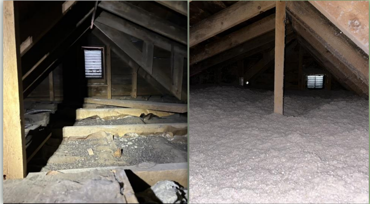
Attic before and after air sealing & insulation
