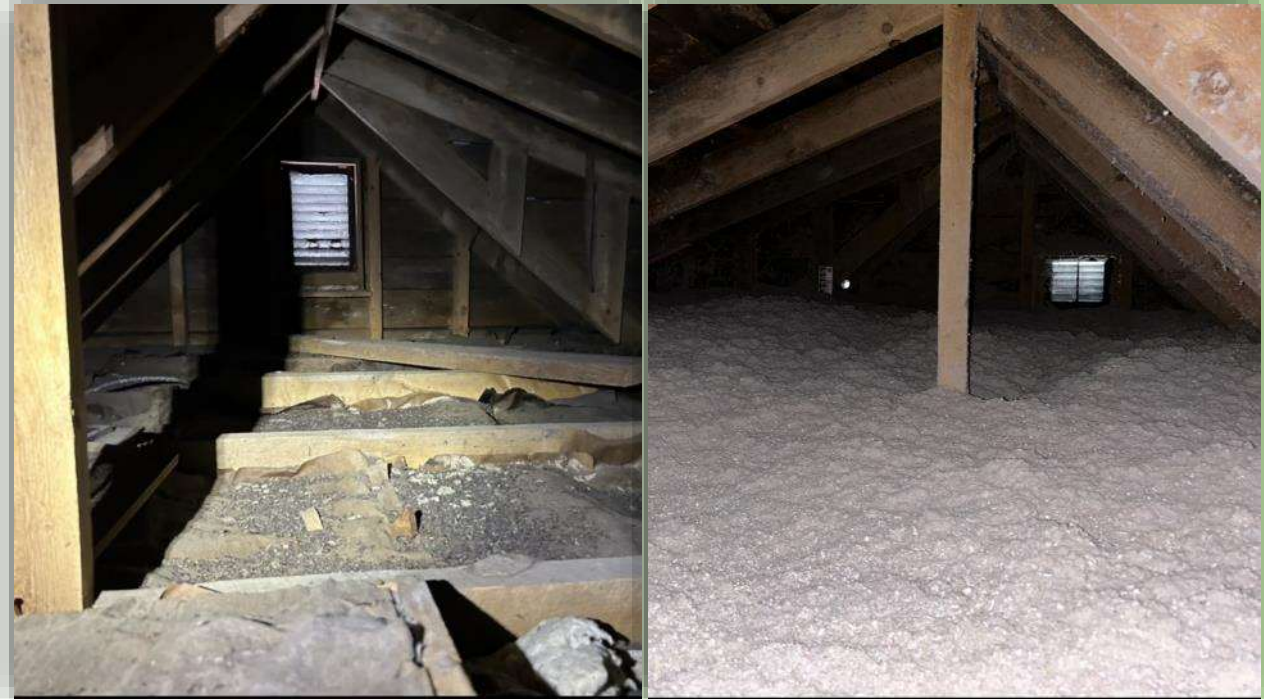
Attic before and after air sealing & insulation
