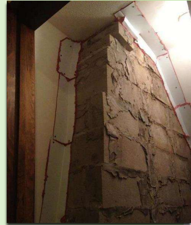
Fire-rated air sealing around an exposed chimney chase
