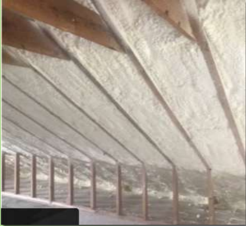
Spray foam prior to drywall fire barrier
