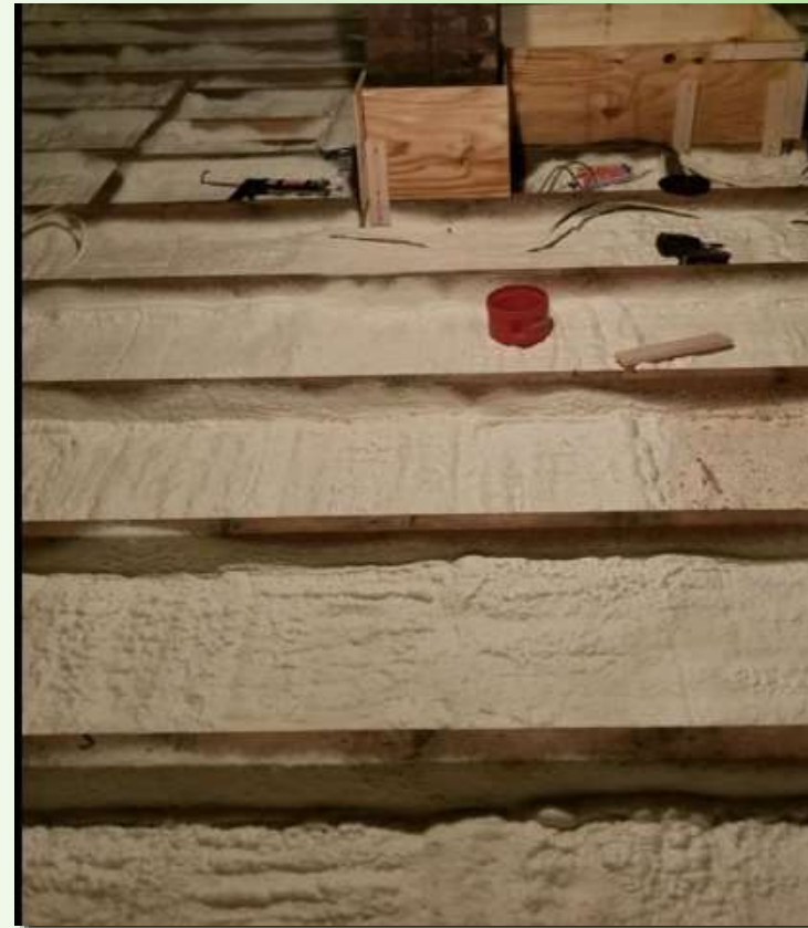
Spray foam "skim coat" attic air seal, prior to insulation
