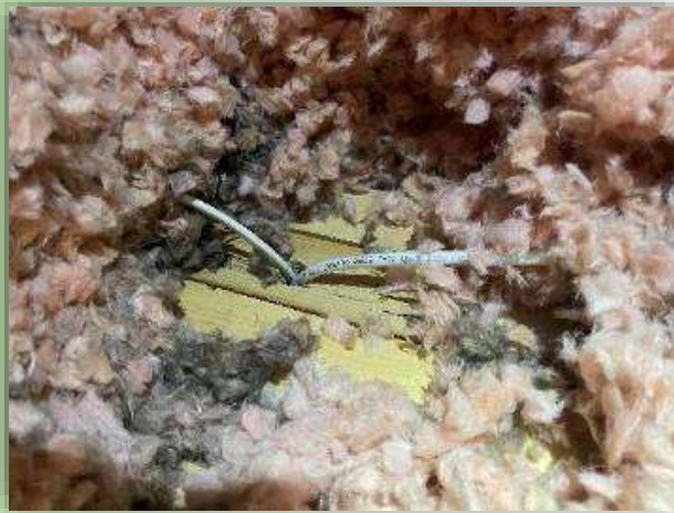
Pipe & electrical penetrations
