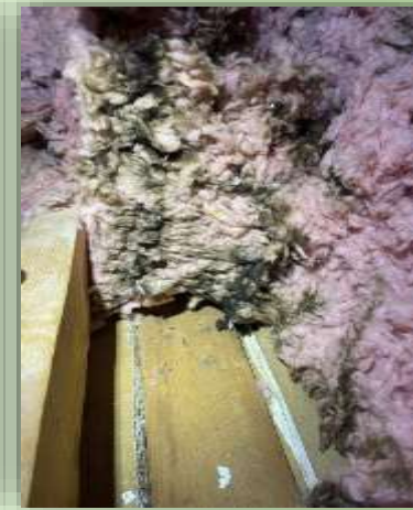
Tops of interior walls
