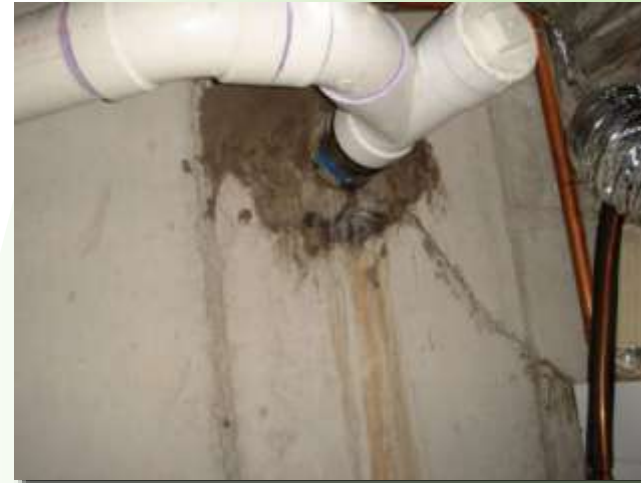
Electrical, plumbing and other penetrations
