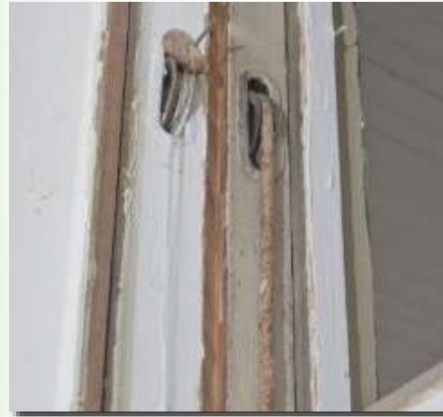
Old pulley-hung windows
